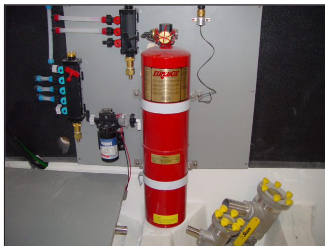
Automatic Fire Extinguisher
