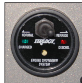
Typical Automatic Fire Extinguisher Monitor Panel
