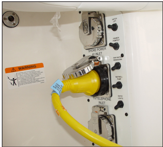
Cockpit Switch Panel and Shore Power, TV and Telephone Inlet Plugs
