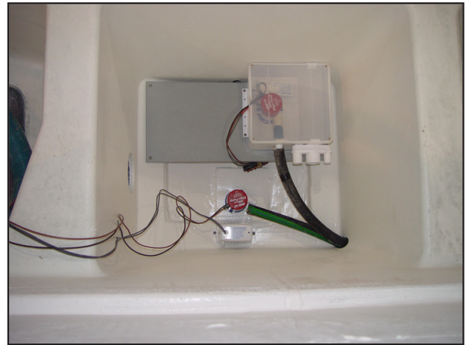
Cabin Drain Sump System and Forward Bilge Pump and Automatic Switch
