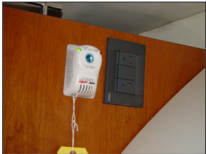
CO Detector and V-Berth GFI and Overhead Light Switch
